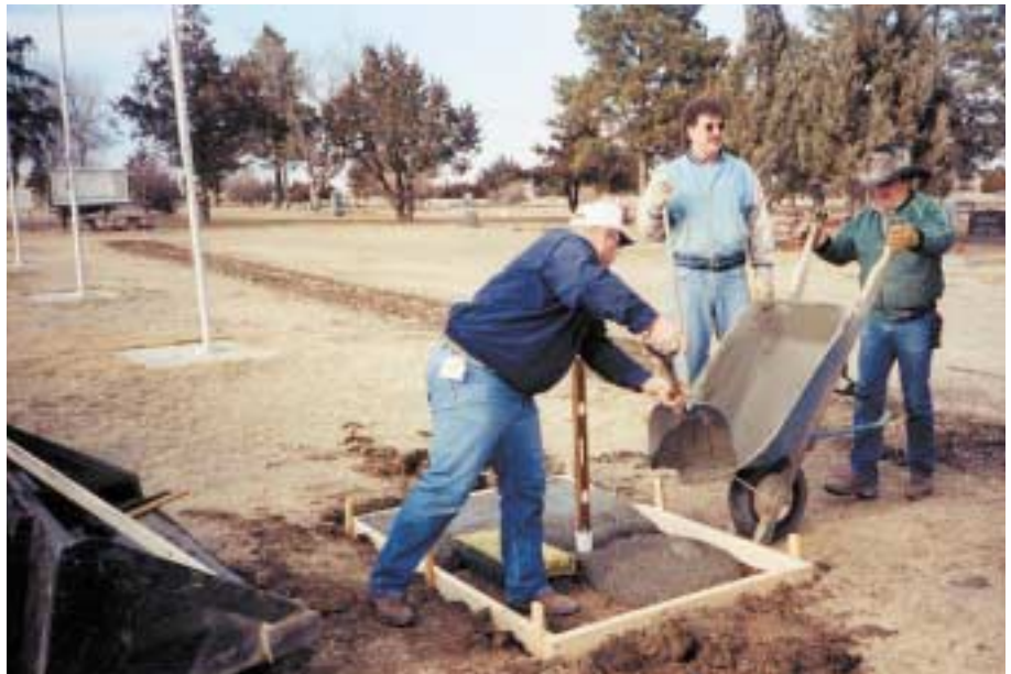
Lester Pearson pours a wheelbarrow full of cement as he, Don Haynes, and Mike Moses install a new flagpole, expanding the row of memorial flagpoles at the entrance of the Philip cemetery.
